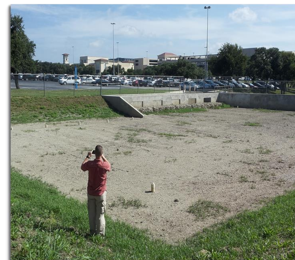
Sand filter basin
